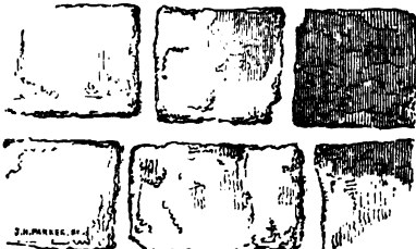
71. Wide-jointed Masonry, Chapel in the White Tower, London, A.D. 1061.
